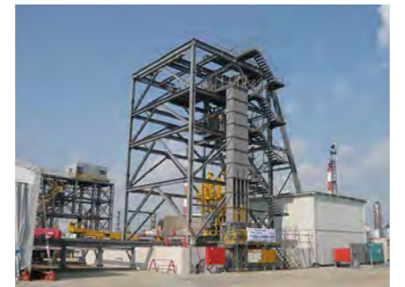
Construction installation for the Natl. LPG Stockpiling Base.
